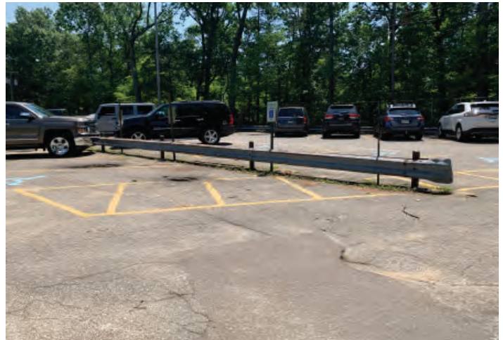
Accessible parking spots are signed but not striped correctly at the Milham Park Golf Course clubhouse.
